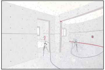
Spray a fog of sealant particles that travels to the air gaps and holes.
