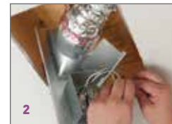
Connect the wiring and attach duct to installation adapter
